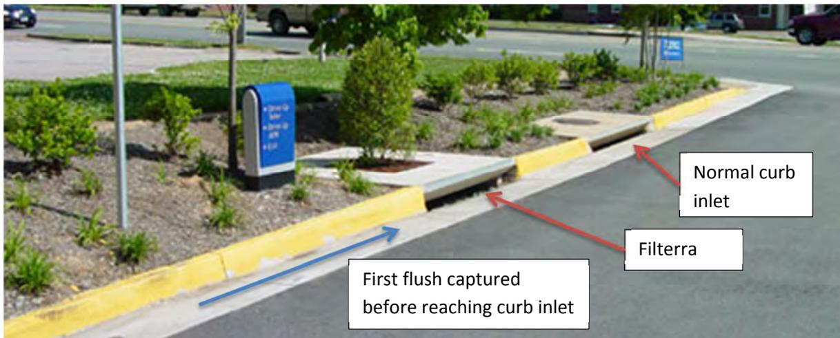
Figure 1 Typical *Filtrerra* installation (Picture from *Filtrerra* website)
