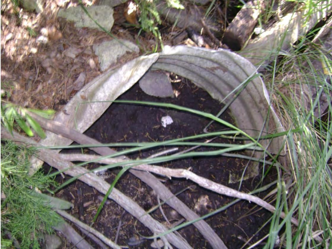
Figure 9 – William Hilton Pkwy drainage system outfall pipe. The pipe is crushed and needs to be replaced.
