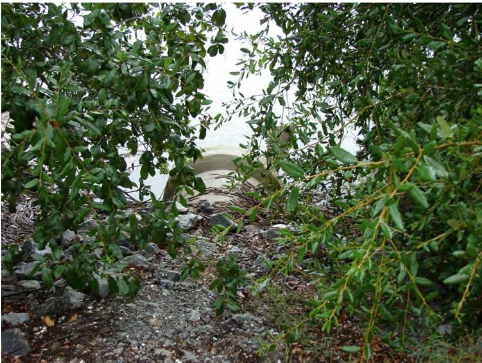
Figure 6 – The discharge end of the pipe needs a backflow preventer to keep saltwater out of the pond and prevent loss of detention volume.
