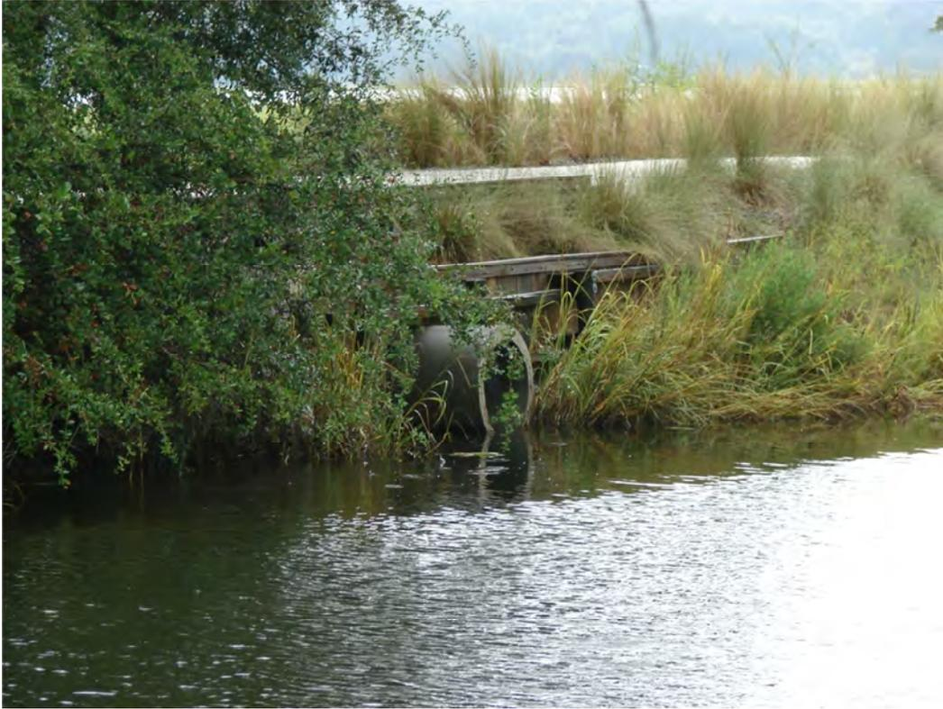
Figure 5 – The existing outlet pipe in the Shelter Cove Park pond does not have a control structure. Retrofitting an outlet structure would improve water quality treatment.
